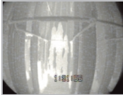
The infrared image above shows the inside of a coal-fired boiler prior to treatment with Fuel Chem. The bright, white areas are slag that has built up on the pipes. Below, the same boiler is shown after only a few weeks of Fuel Chem treatment. Note almost no white areas depicting slag in that image.
