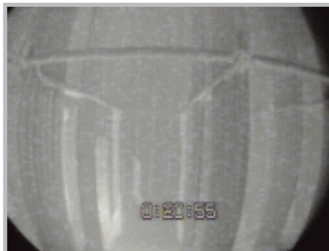
The infrared image above shows the inside of a coal-fired boiler prior to treatment with Fuel Chem. The bright, white areas are slag that has built up on the pipes. Below, the same boiler is shown after only a few weeks of Fuel Chem treatment. Note almost no white areas depicting slag in that image.
